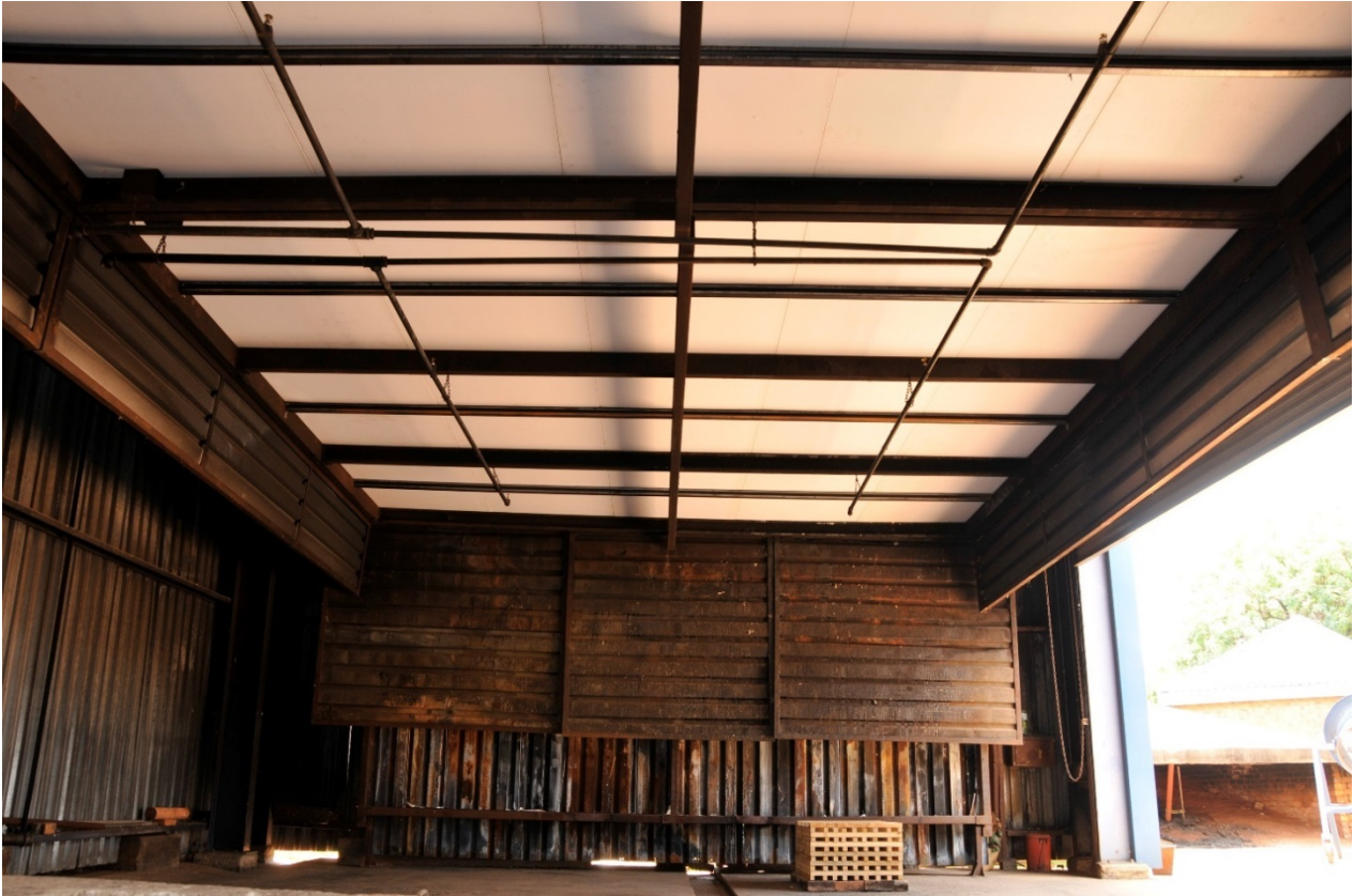
Figure 4.1: The SANS 10177 – 11 test installation prior to ignition of the Fire Source
