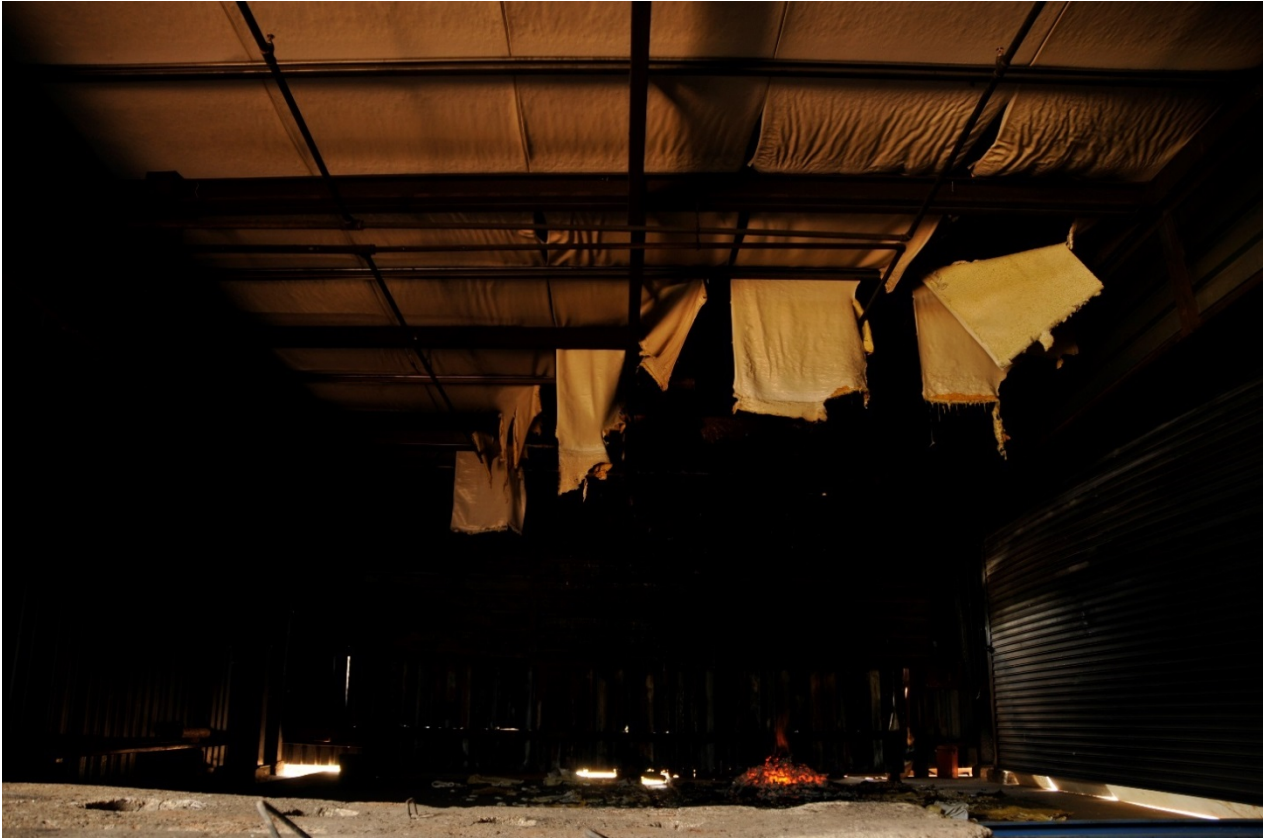
Figure 4.11: Test installation at conclusion of test
