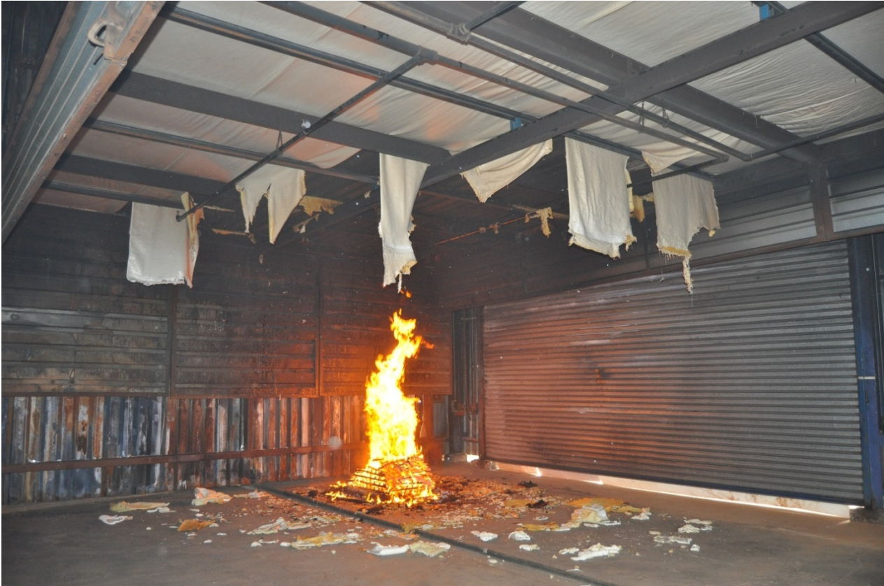
Figure 4.9: Debris dropped down up to 3 rd bay (4 - 6 m distance)
